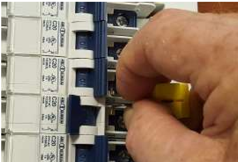
FIG 2 STEP 2 – APPLYING LOCKOUT
