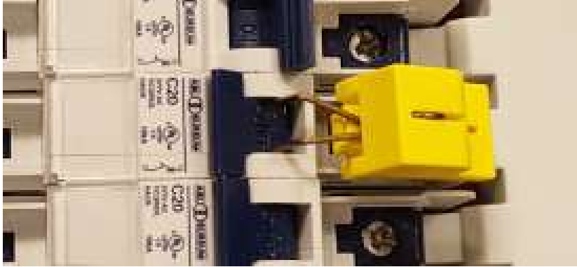
FIG 2 STEP 3 – LOCKOUT ATTACHED
